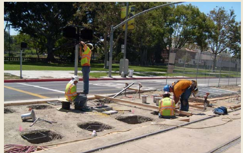
Sidewalk reconstruction (t) and installation of Bollards (b) at Trousdale Parkway
