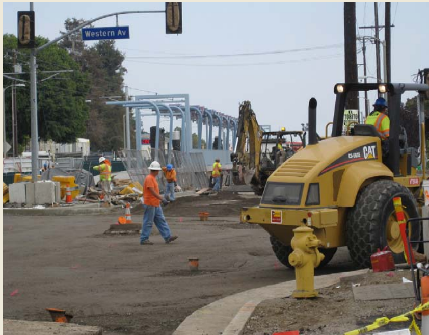
Reconstruction/restoration work at Western Ave
